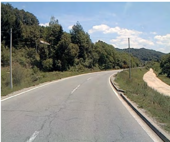
Figure 5: A steep slope, trees and electric pole in the roadside area
