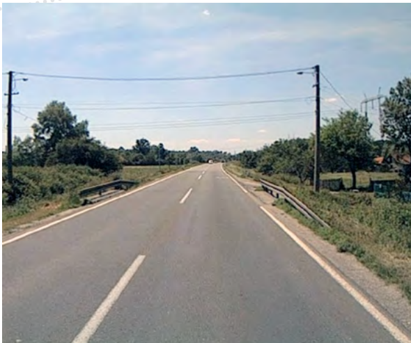
Figure 3: Unsafe ends of safety barriers, canal, electric pole in the roadside area
