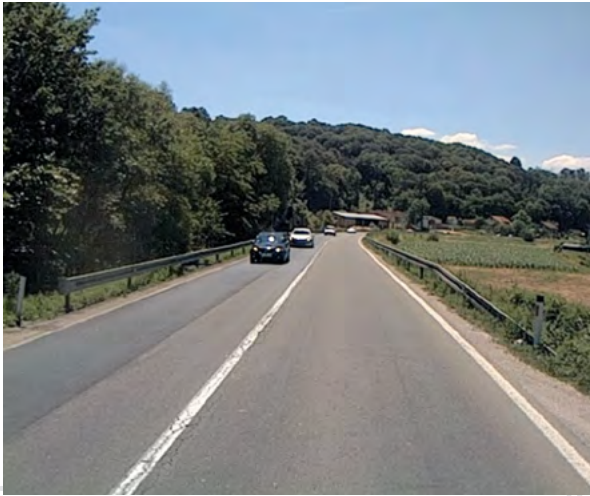
Figures 1 and 2: Unsafe ends of safety barriers
